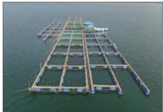
Cages Installed in Kasarsai Reservoir
