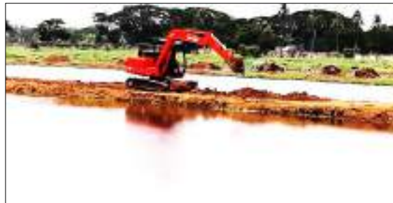
Earthwork of bunds at NFFBB pond
