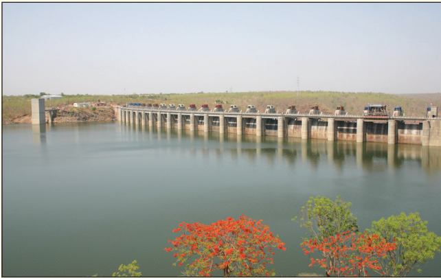
Indira Sagar Dam across river Narmada in Khandwa district of Madhya Pradesh State
